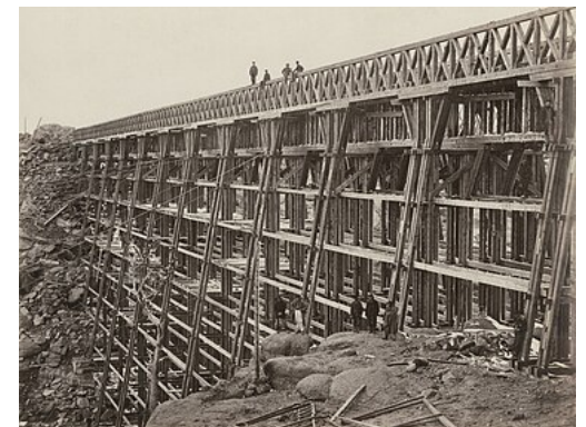
Dale Creek Bridge
